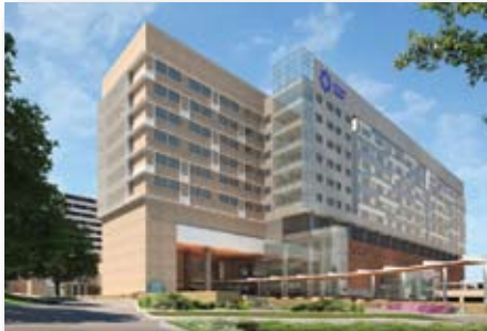
Tower at University Hospital
